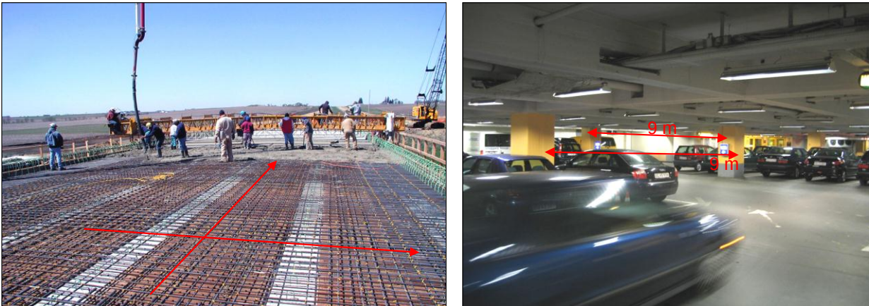
Figure 1.2. Reinforcement arrangement for a double span bridge deck (left) and double spanning slabs in a parking garage at Illums Bolighus (right).
